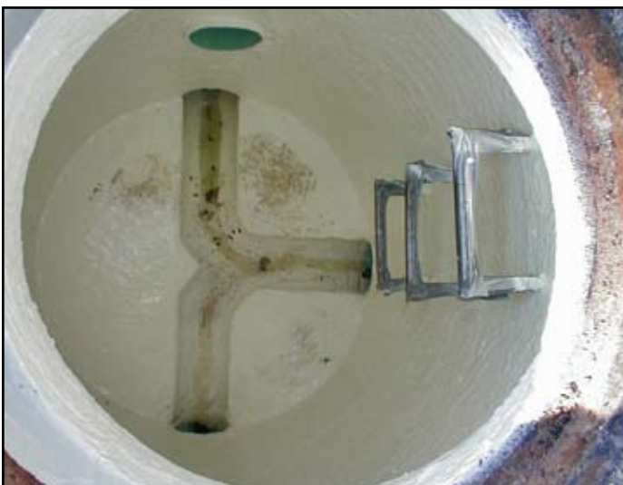
Monolithic lined manhole.
