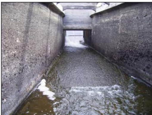
Flume before work commenced.
